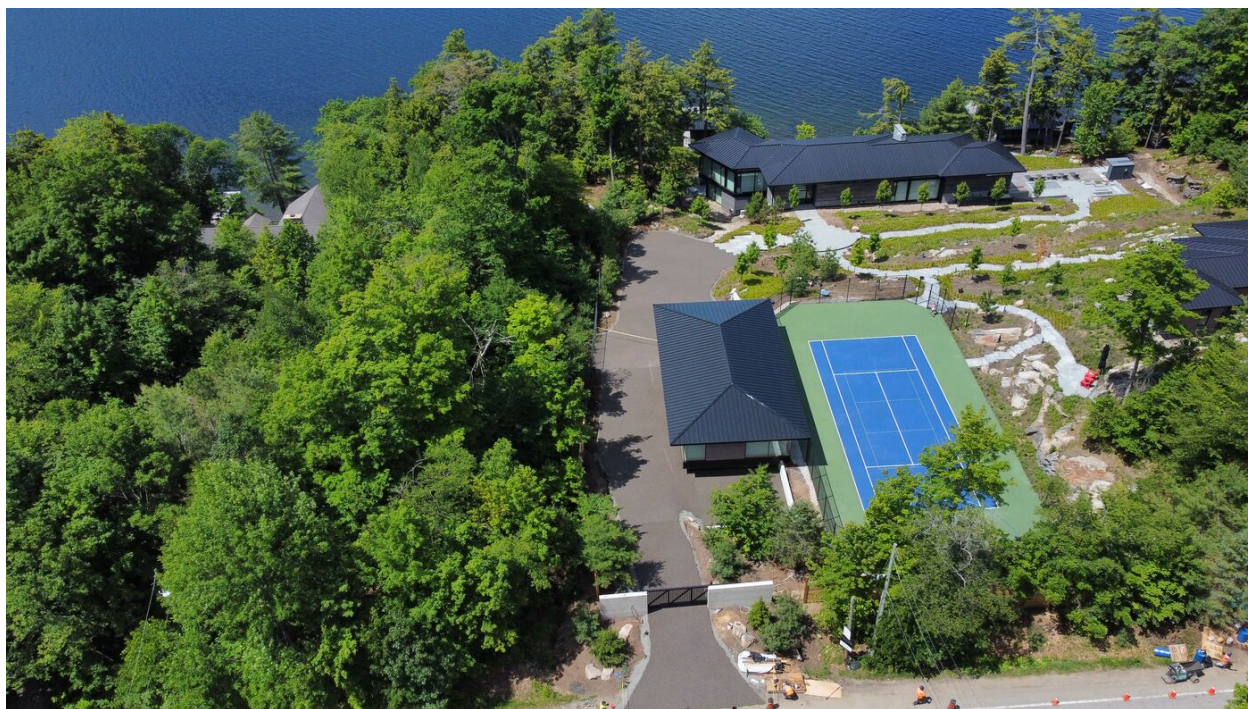
Aerial view of the completed 700m² driveway winding through the Muskoka property to the water's edge.
