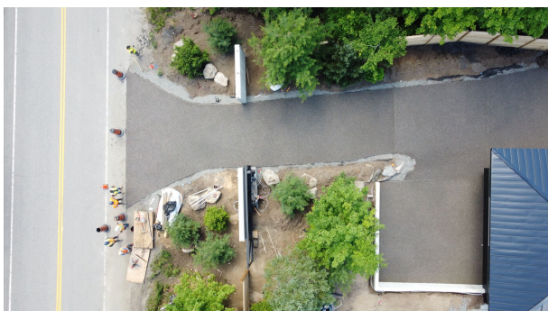
Dream Pavé's crew shaping the curved path sections ahead of final grading and planting.
